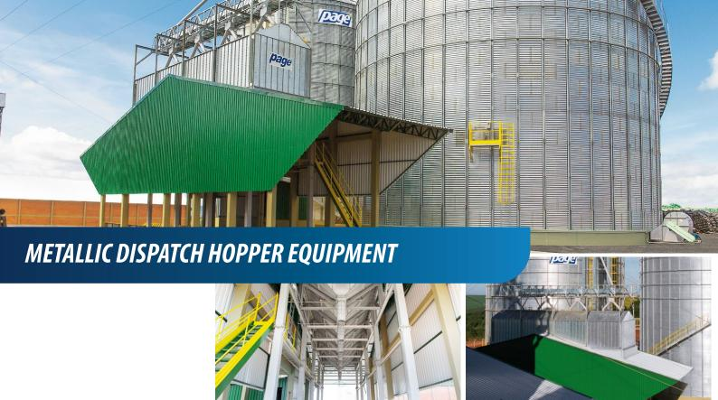
The metallic dispatching hopper Pagé has its body manufactured in galvanized panels with internal reinforced beams. They are modeled in 4X4 meters cells, each one having the storage capacity of 40 tons for products as soybean, corn, wheat, sorghum and others.
